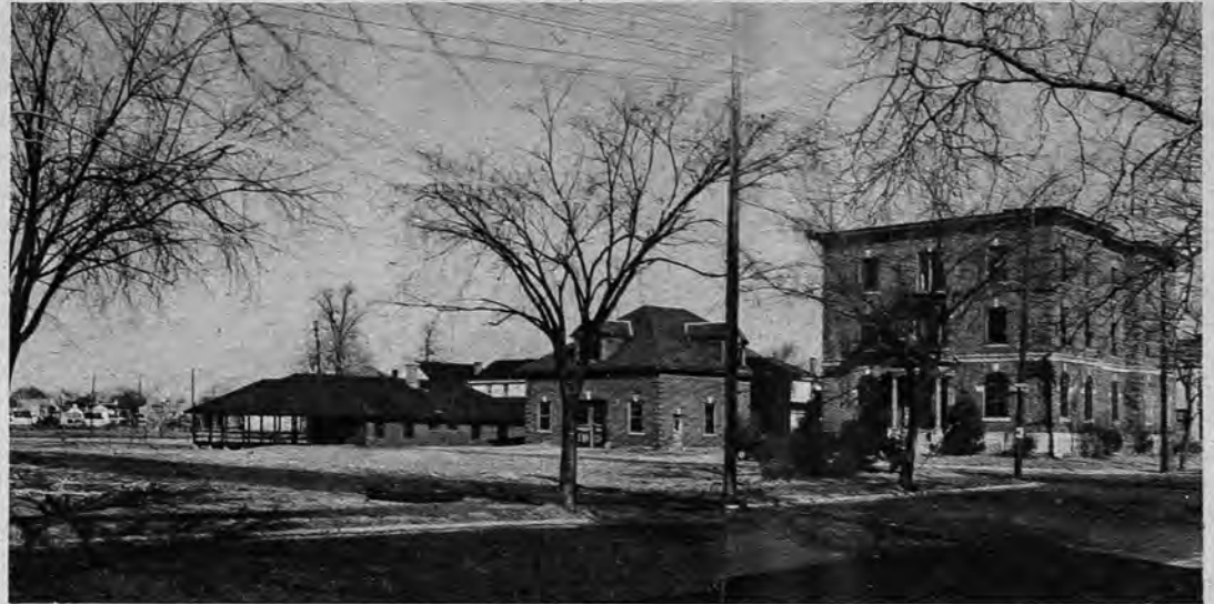
The above photograph shows the buildings located on Sessions Street in which the Center is interested. It is the location of the old Sessions Street Police Station.
