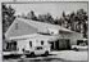
The new 100,000-sq-ft building will house the camp's administrative offices, a dining hall, a recreation center, and a gymnasium.
