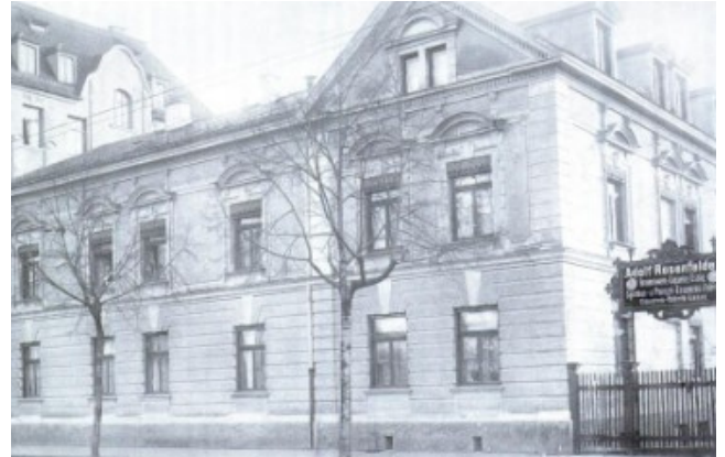
The Regensteiner and Aufhäuser house at Hermanstrasse 23 in Augsburg, Germany, with the entrance to the Adolf Rosenfelder company to the right.
